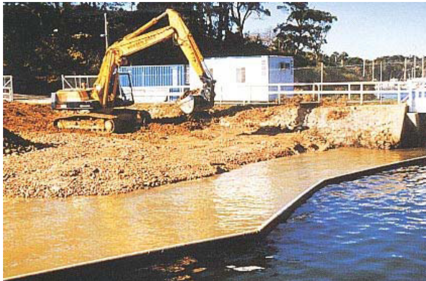
Floating Silt Curtain (Courtesy of Geofabrics Australasia)
