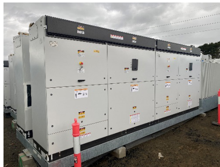
Photo 20 Power Conversion Units (PCUs) awaiting installation (painted mild grey) (4 May 2022)
