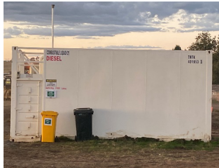
Photo 28 Self-bunded diesel storage tank (4 May 2022)
