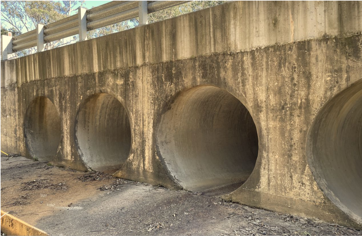
Figure 4.14-1 Four Pipes at Ch42400
