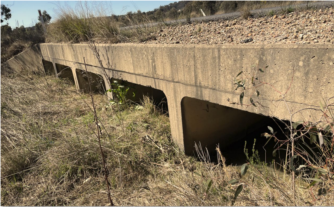
Figure 4.8-1 Five single-cell culverts at Ch30400
