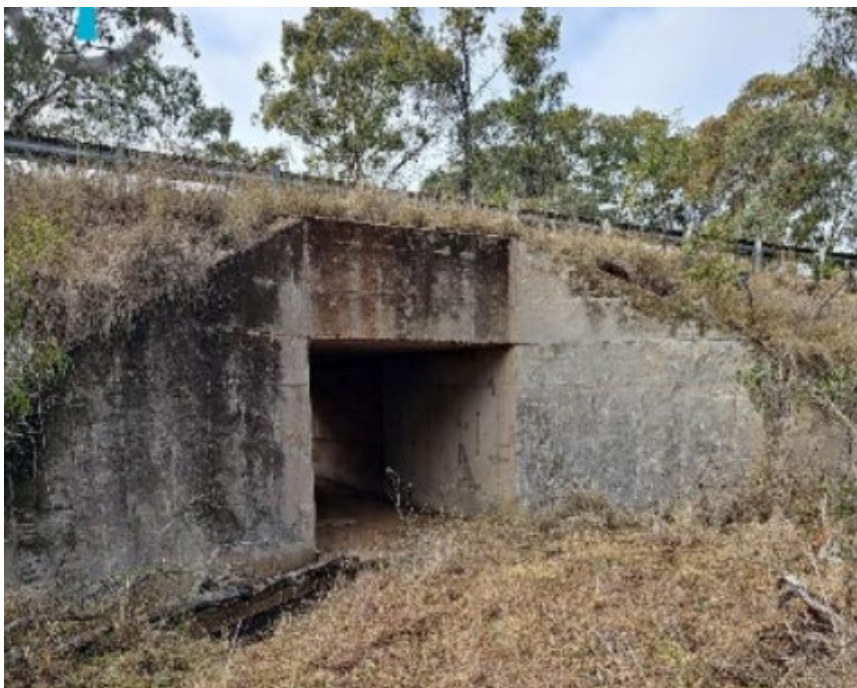
Figure 4.3-1 Single -cell culvert at Ch16600
