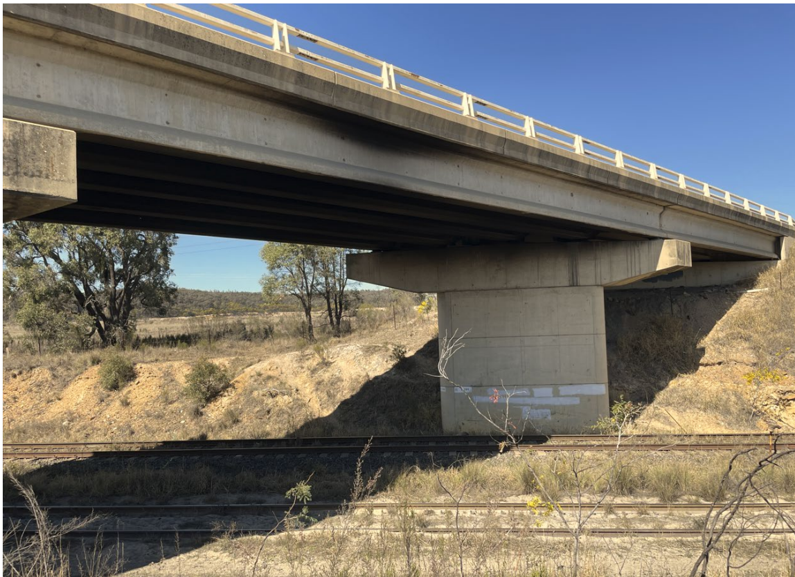
Figure 4.7-1 Bridge over Sandy Hollow-Ulan Railway at Ch29400
