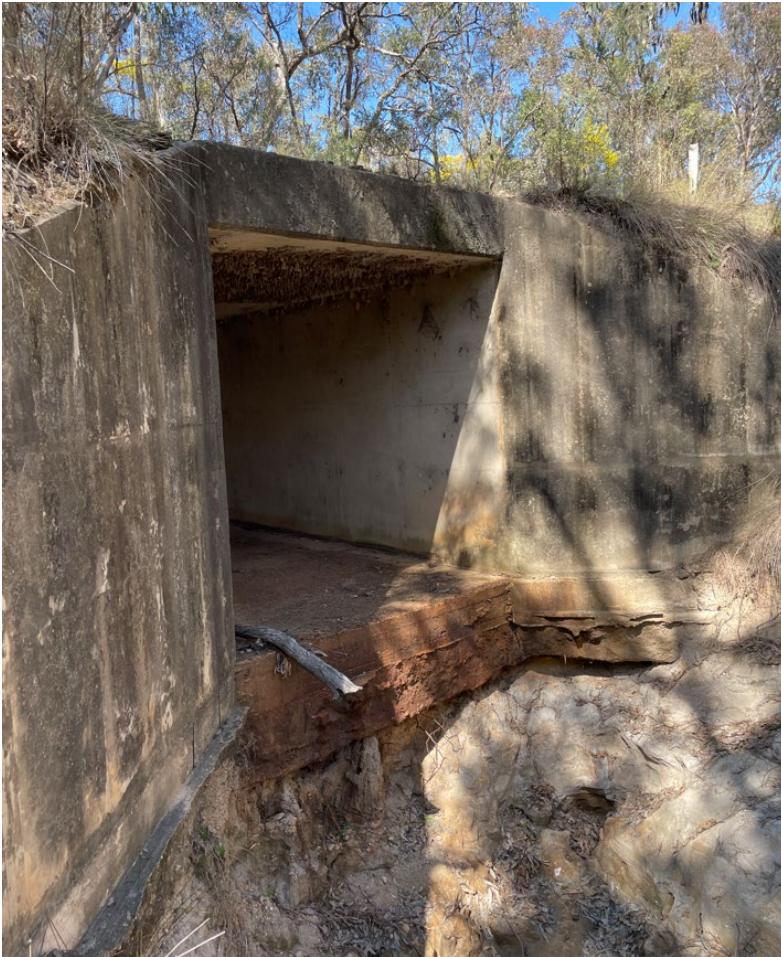
Figure 4.6-1 Single-cell culvert at Ch24300
