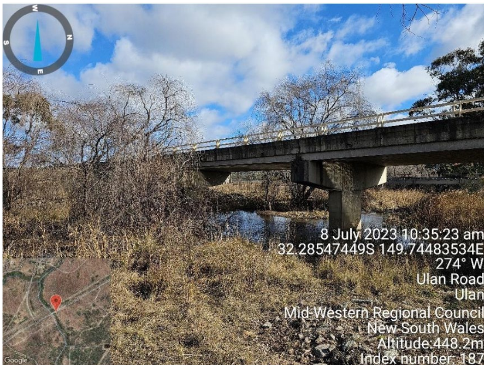
Figure 4.9-1 Bridge over Sandy Hollow-Ulan Railway at Ch32500
