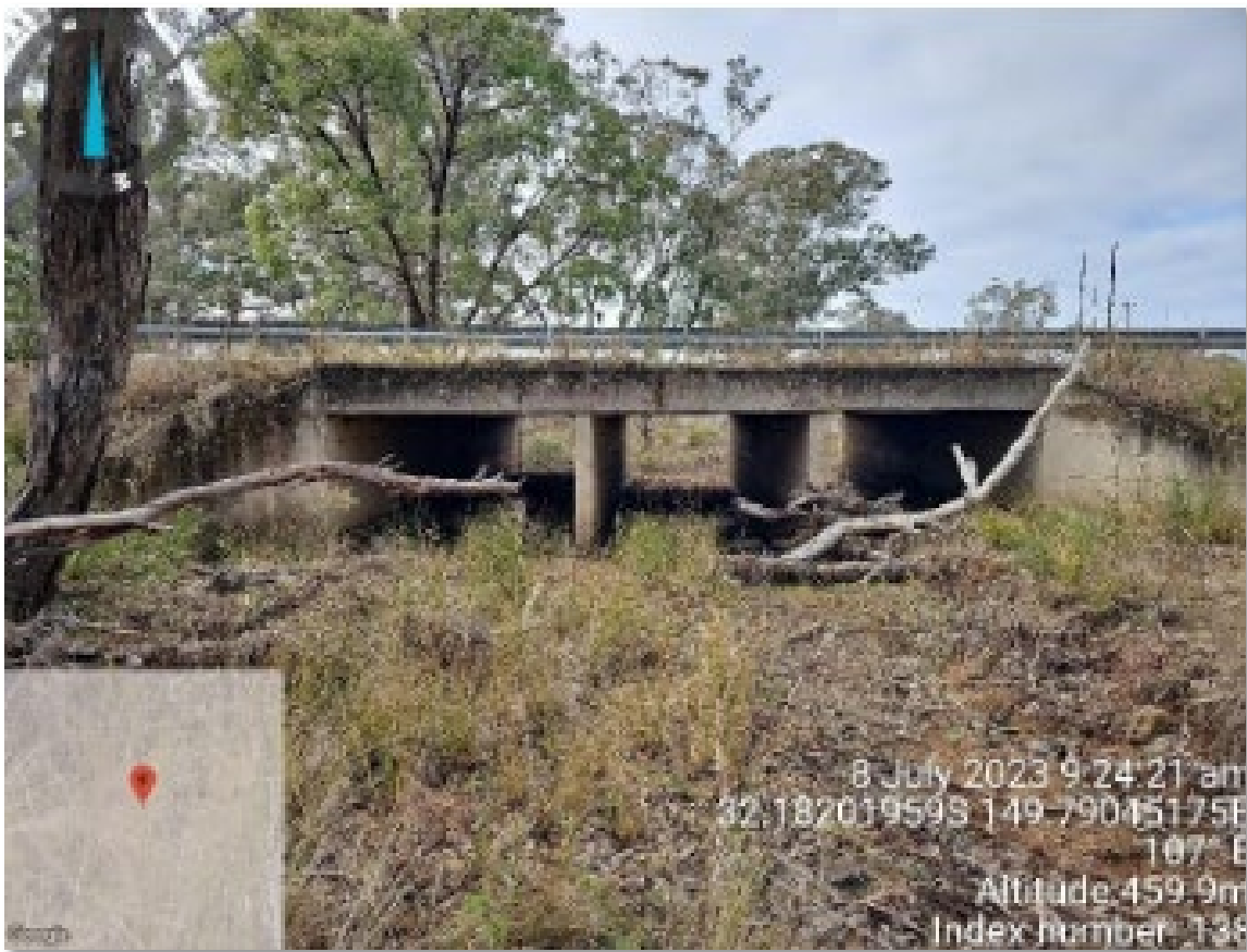
Figure 4.4-1 Three -cell culvert at Ch18600
