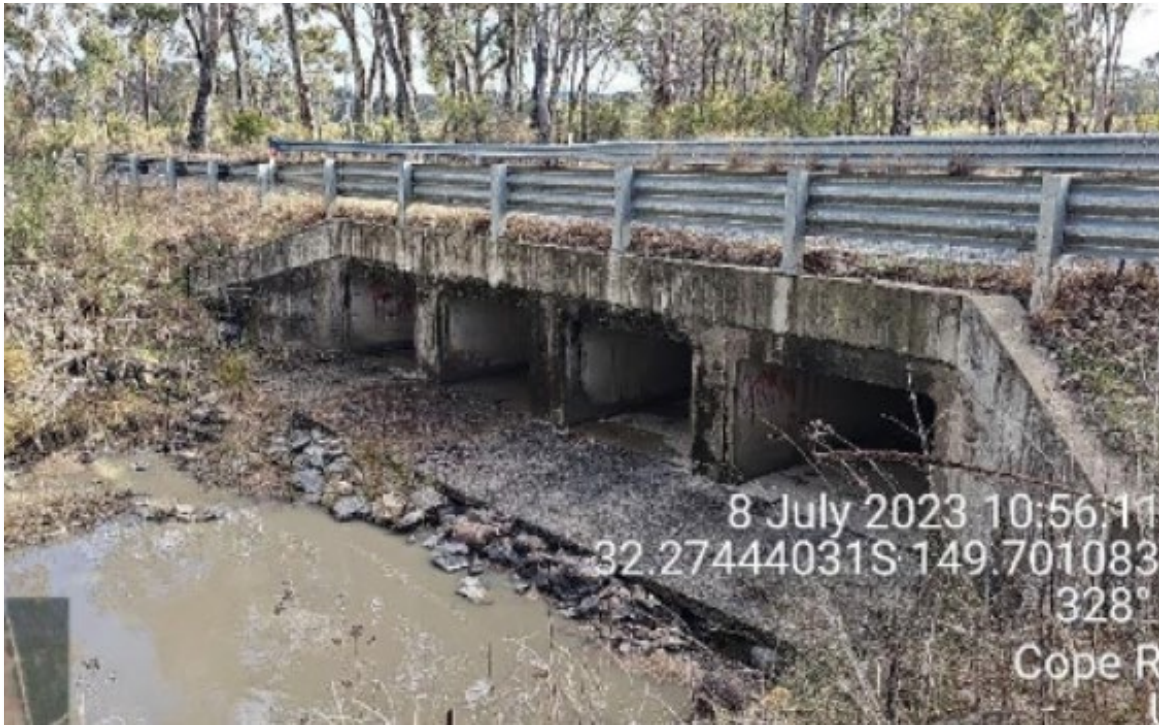
Figure 4.12-1 Four single-cell culverts at Ch37900
