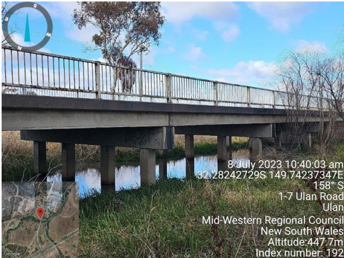
Figure 4.10-1 Bridge over Sandy Hollow-Ulan Railway at Ch33300
