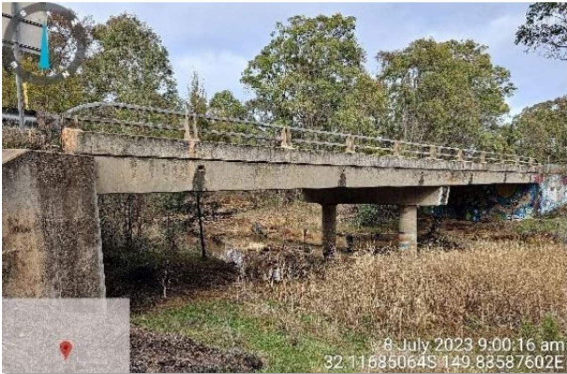
Figure 4.1-1 Murrumbline Creek Turill Bridge at Ch9500
