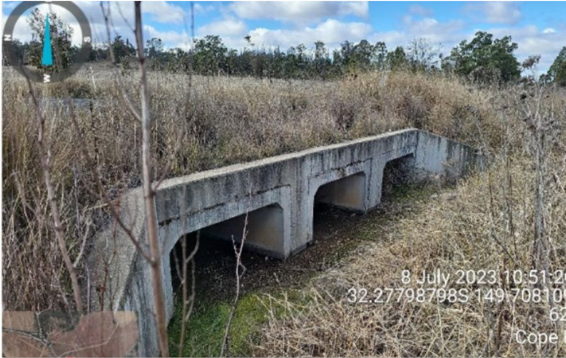
Figure 4.11-1 Three single - cell culverts at Ch37200
