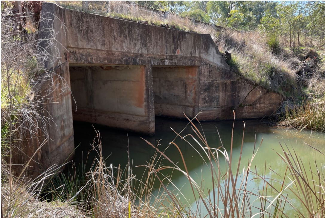
Figure 4.2-1 Twin-cell culvert at Ch12500
