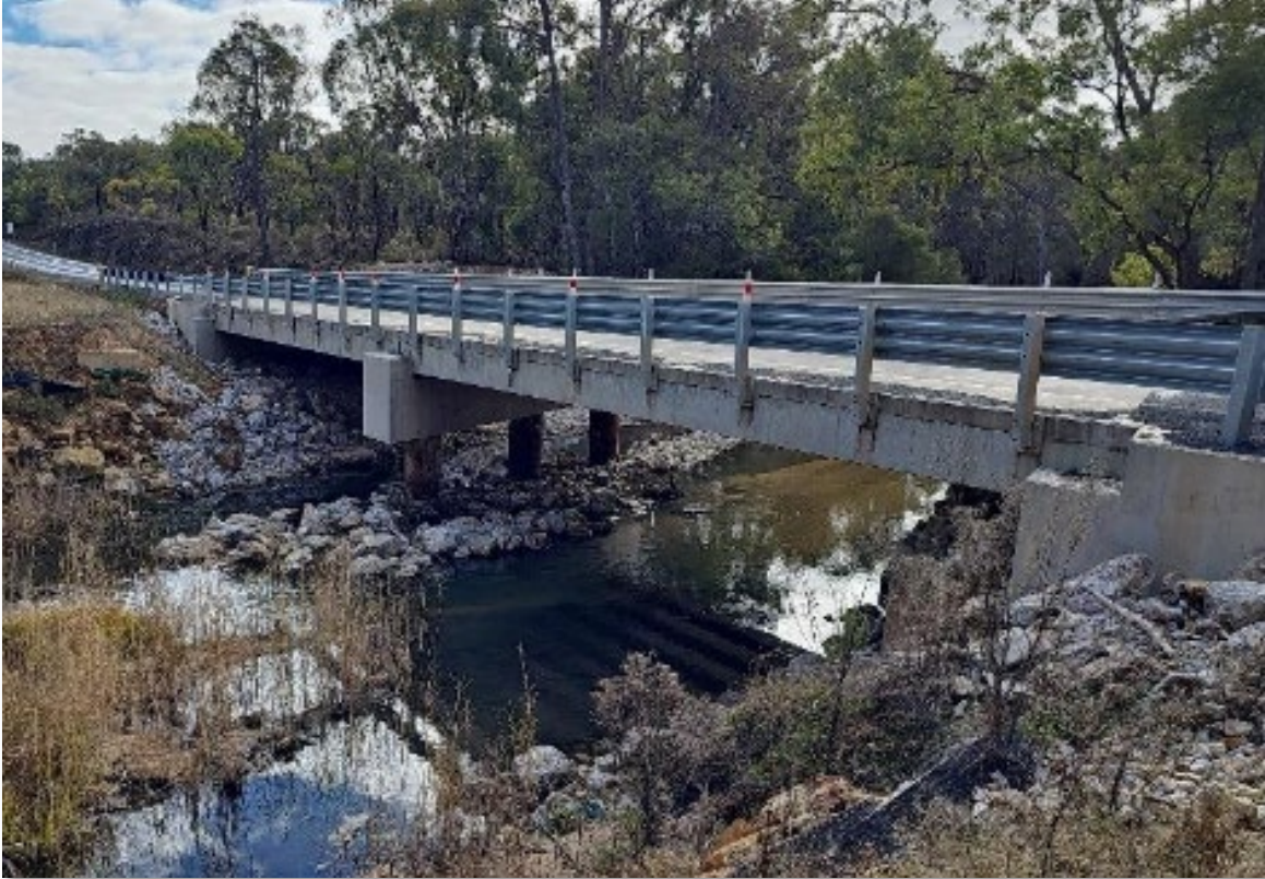
Figure 4.5-1 Bridge over Goulburn River at Ch22700
