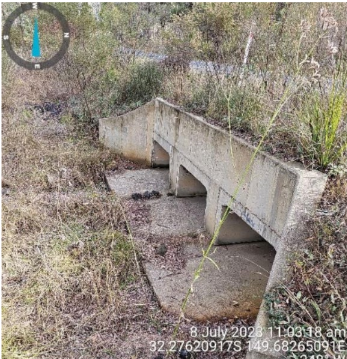
Figure 4.13-1 Three single-cell culverts at Ch39700
