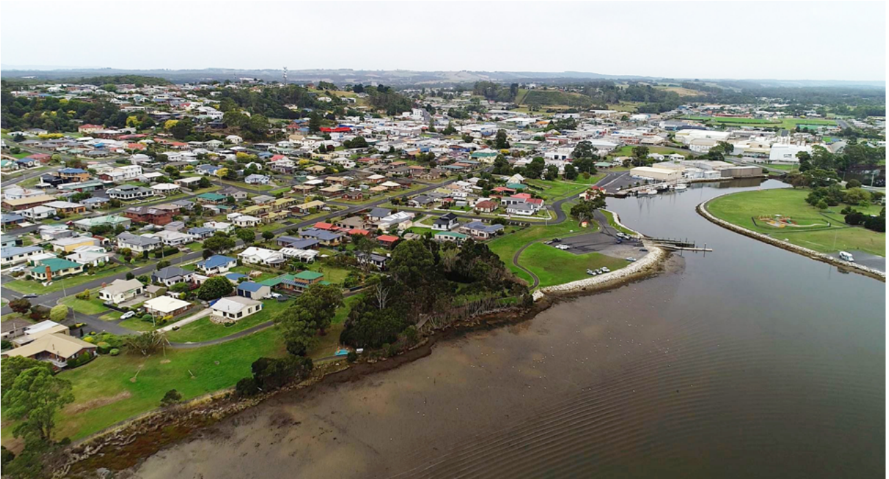
The township of Smithton.
