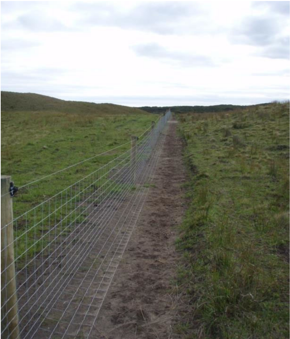
Figure 2 Wallaby-proof fencing installed on Robbins Island
